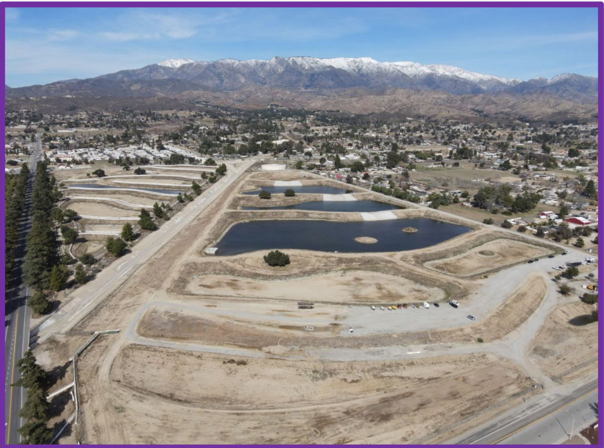
BCVWD Recharge Facilities
