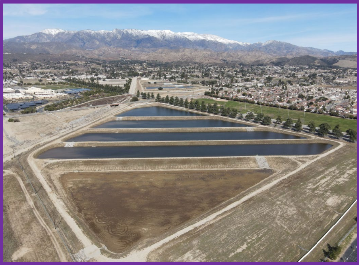
Brookside East Recharge Facility
