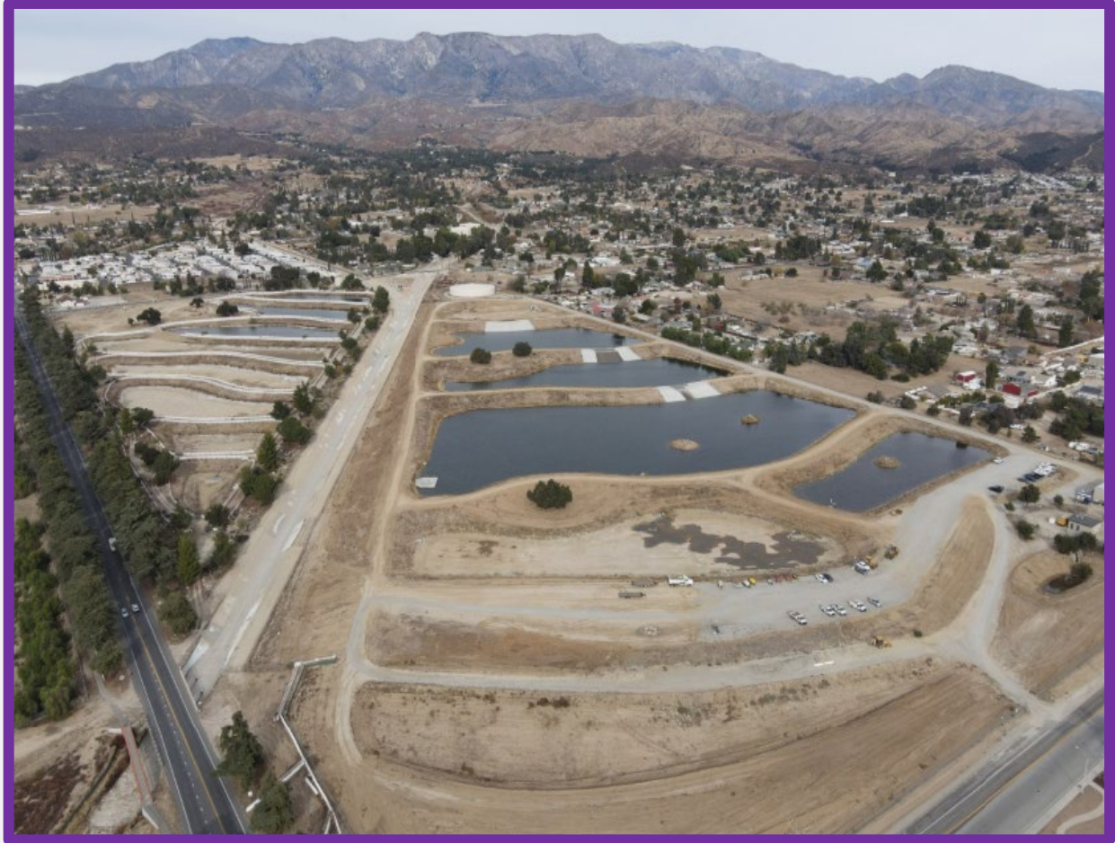
BCVWD Recharge Facilities
