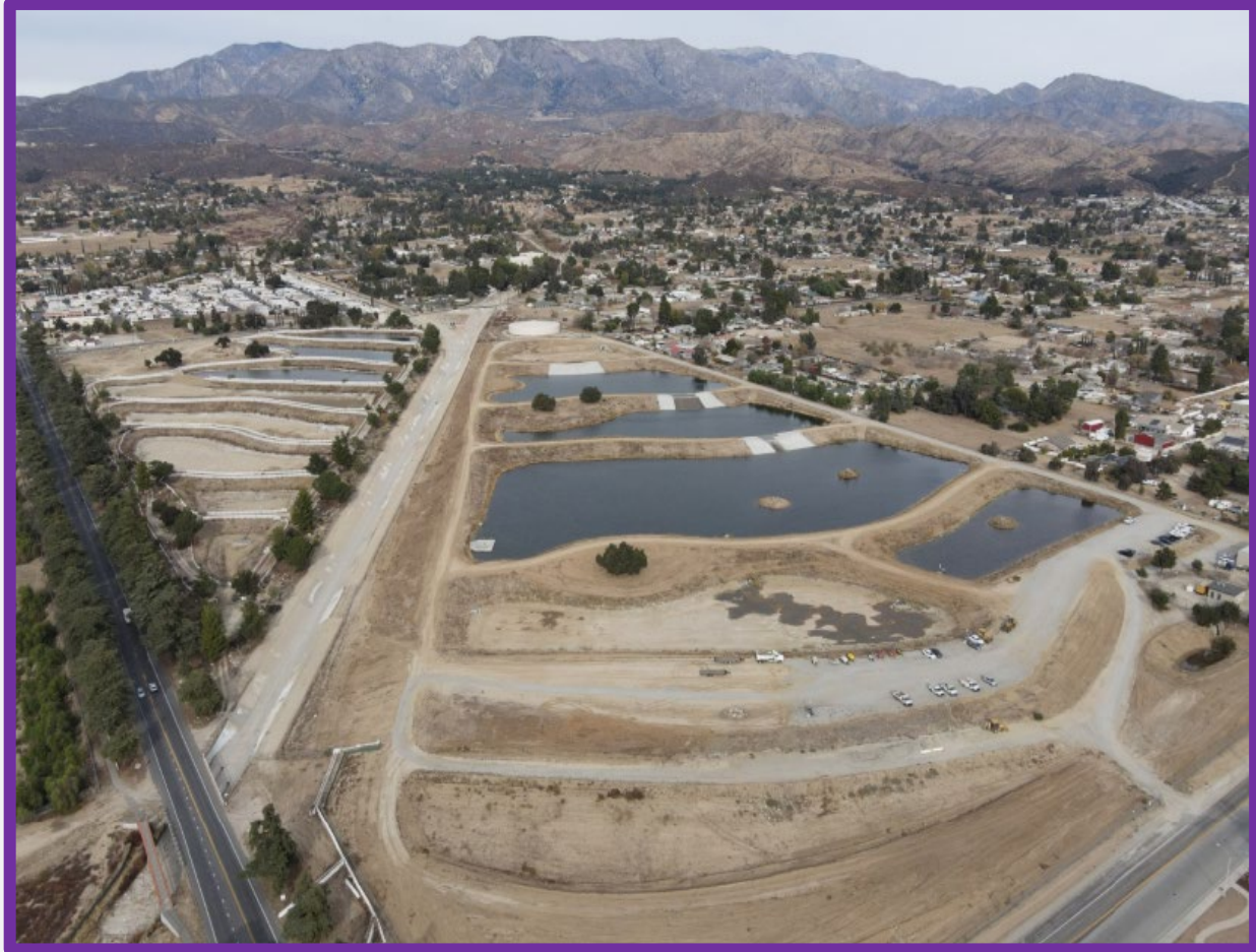
BCVWD Recharge Facilities
