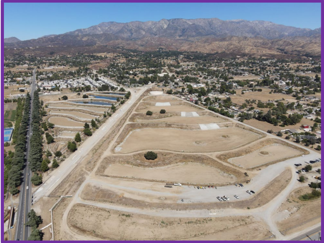
BCVWD Recharge Facilities
