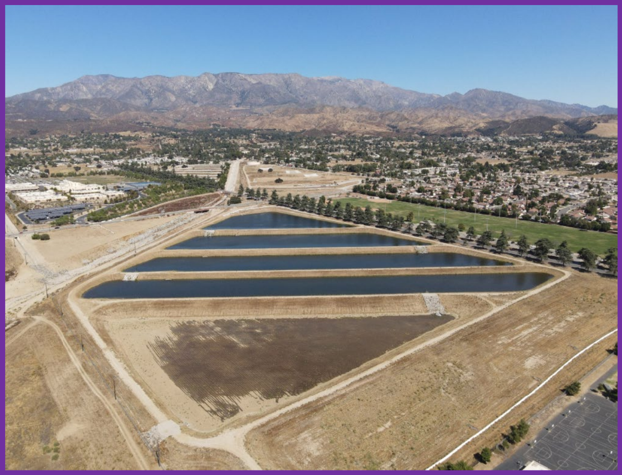
Brookside East Recharge Facility
