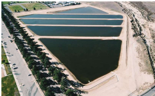
Brookside East Recharge Facility
