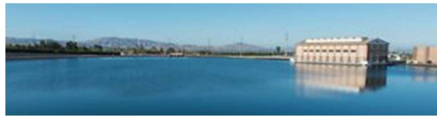
Citrus Reservoir and Pump Station
