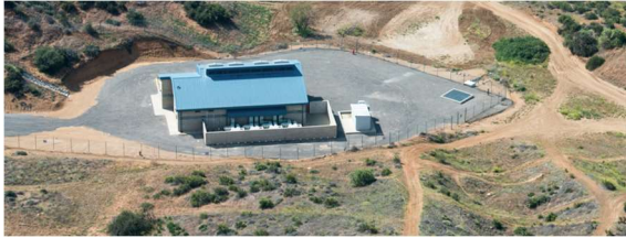
Cherry Valley Pump Station
